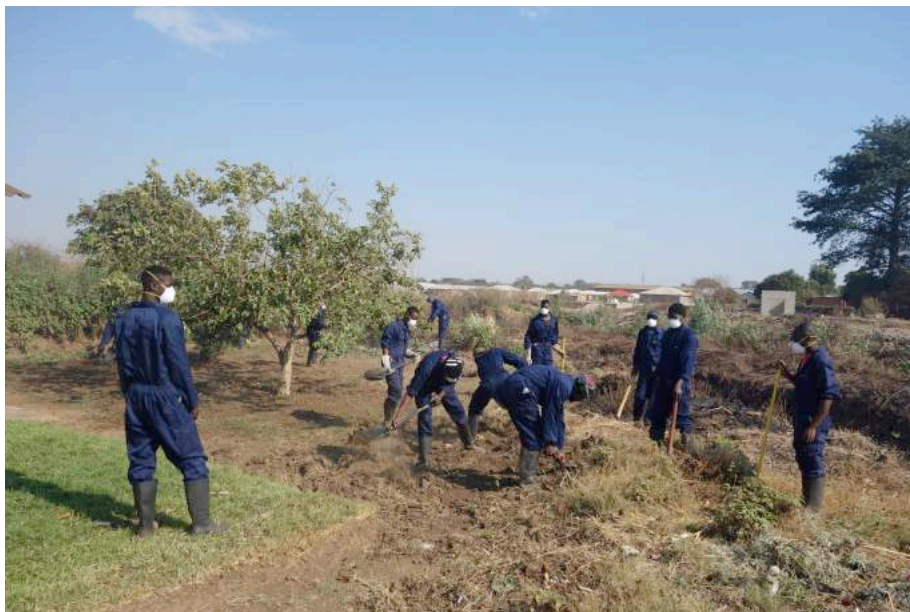
Above: One of several remediation teams prepares a yard for encapsulation with a barrier cloth
