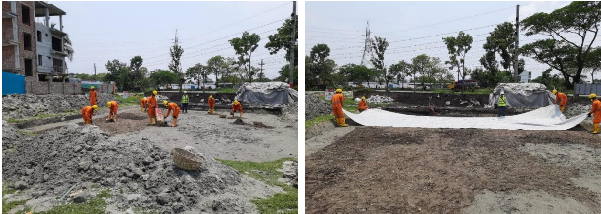
Figure 41: Placing scrapped contaminated soil and geotextile marker layer in the South dumping site.
