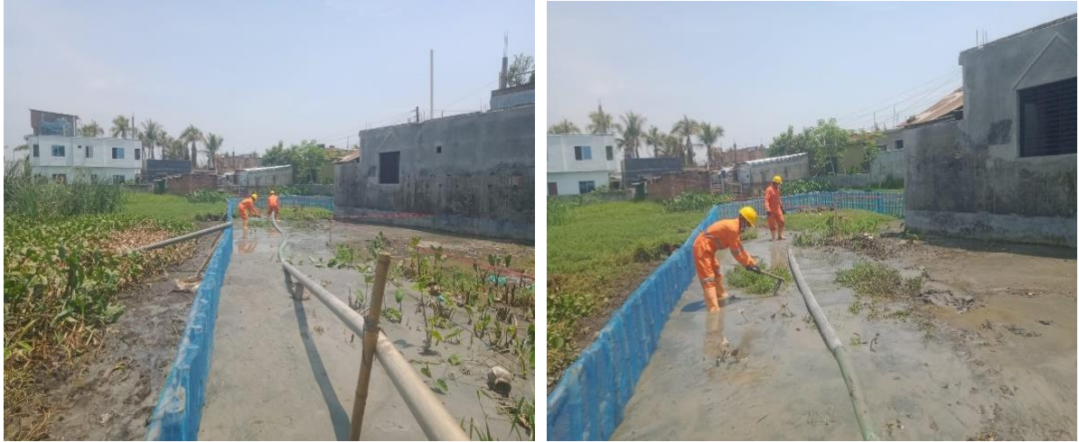
Figure 22: Sand filling of the North and West dumping sites.
