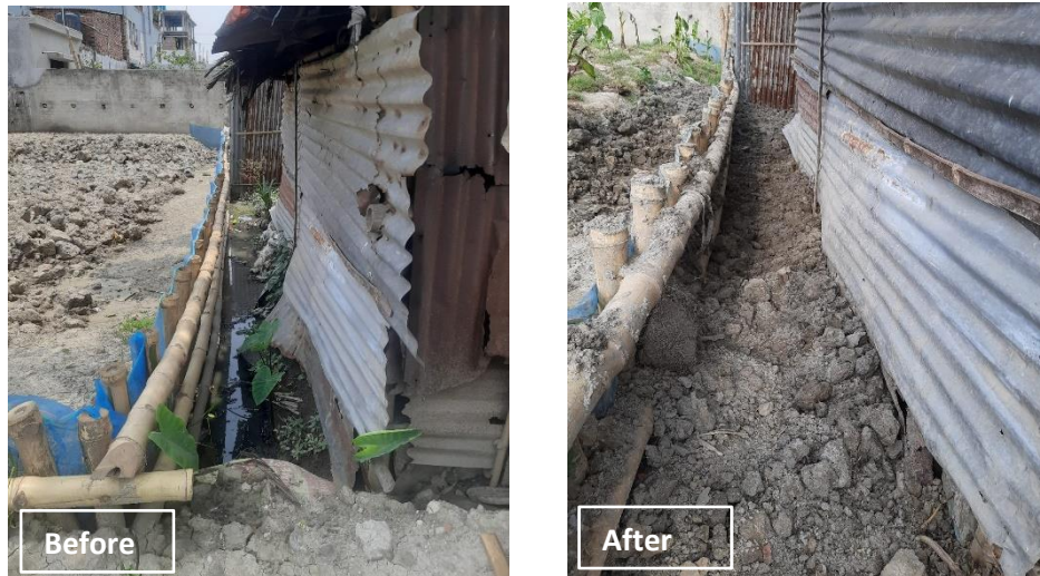
Figure 53: Waterlogging issue due to the capping work in the South site of the West dumping site.
