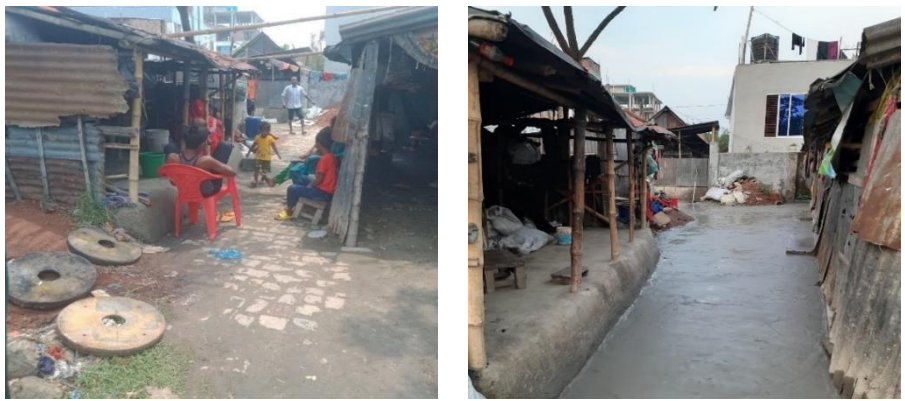
Figure 33: Road and house yard brick soling area before (left) and after (right) concrete work.
