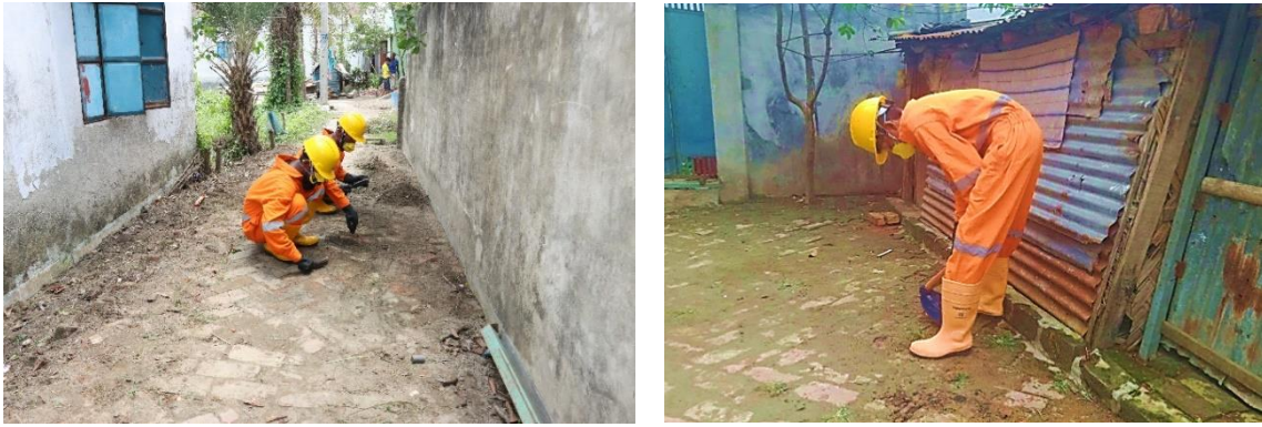
Figure 30: Scraping of soil from brick soling road and yard areas.
