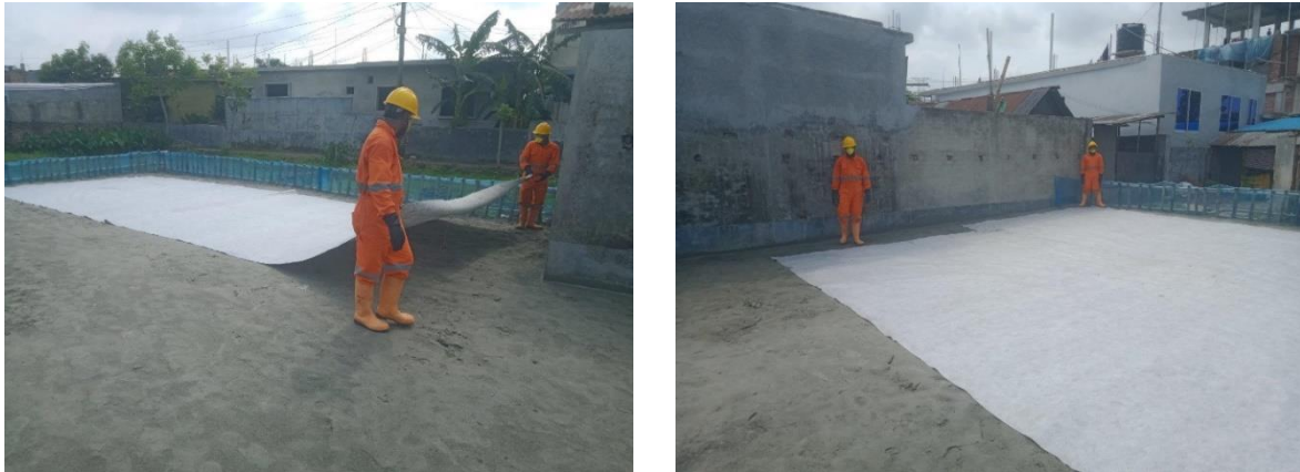
Figure 24: Placing geotextile layer in the North and west dumping sites.
