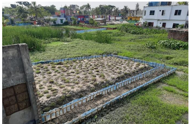
North dumping site after remediation work
