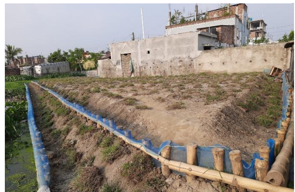
West dumping site after remediation work
