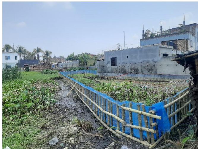
Figure 21: Bamboo piling work in the North and West side of Mr. Badi's house.
