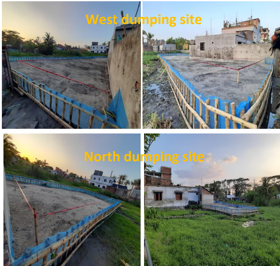
Figure 23: North and West side dumping sites after 1 ft sand filling
