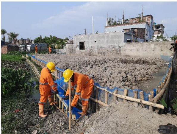
Figure 27: Bamboo piling with 1:1 slope and placing grass at North and West dumping site.
