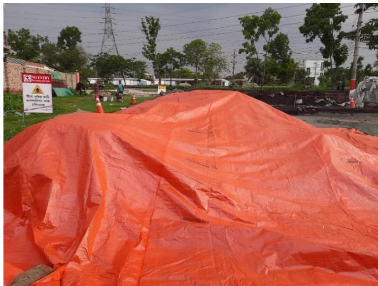
Figure 40: Tarpaulin was used for covering the excavated clean sand stockpile of the south dumping site.
