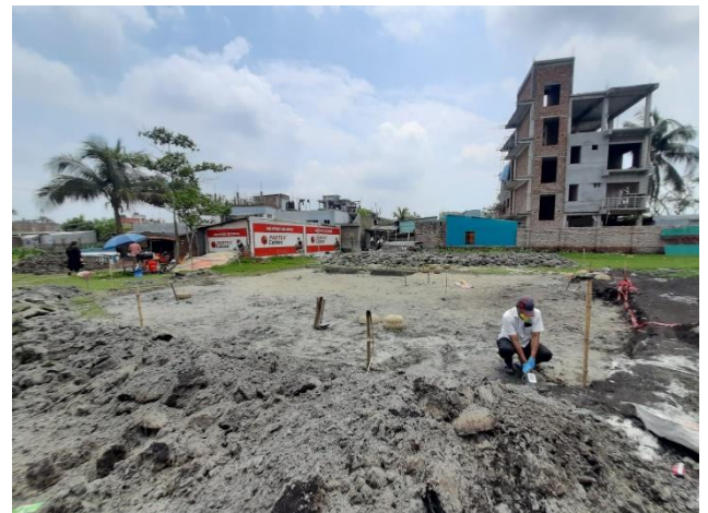
Figure 36: Excavation of top 1 ft soil of the south dumping site.
