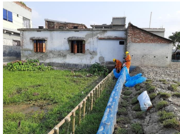
Figure 27: Bamboo piling with 1:1 slope and placing grass at North and West dumping site.
