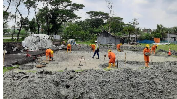
Figure 36: Excavation of top 1 ft soil of the south dumping site.
