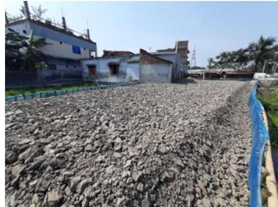
Figure 26: Placing clean soil and 1:1 slope work at North and West dumping site.
