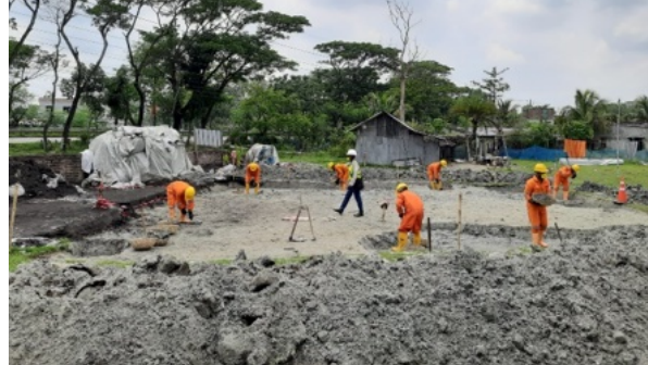
Figure 36: Excavation of top 1 ft soil of the south dumping site.
