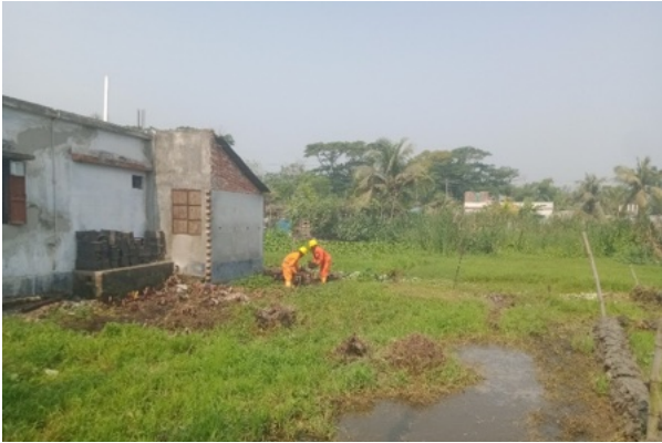
North dumping site before remediation work
