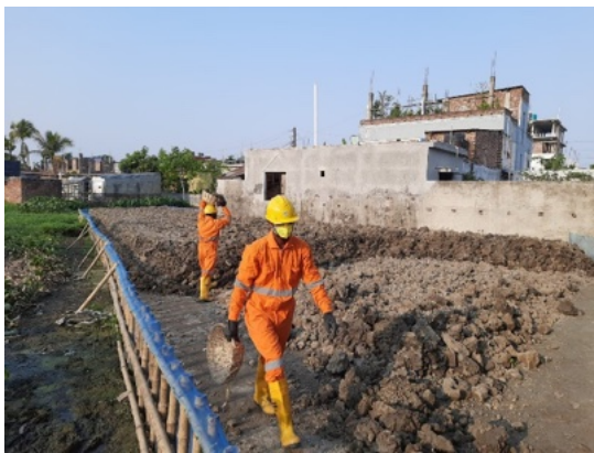
Figure 26: Placing clean soil and 1:1 slope work at North and West dumping site.
