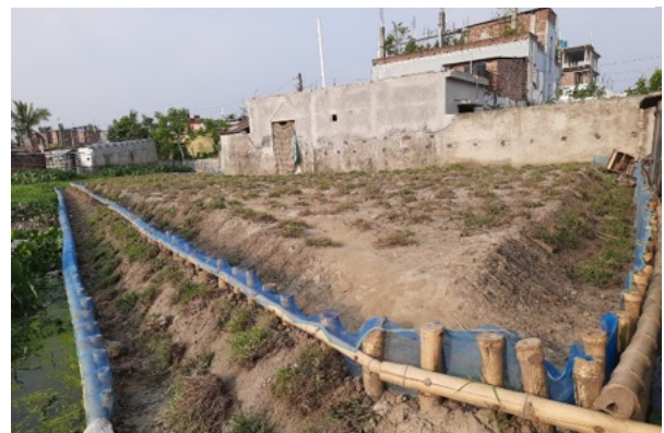
West dumping site after remediation work
