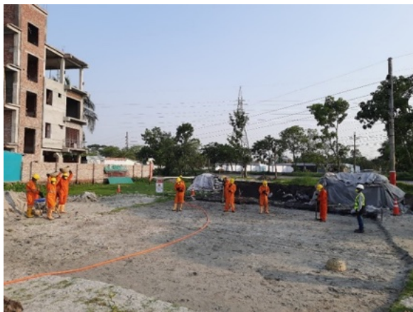
Figure 42: Filing south dumping site with 1 ft excavated sand and 1ft clean soil.
