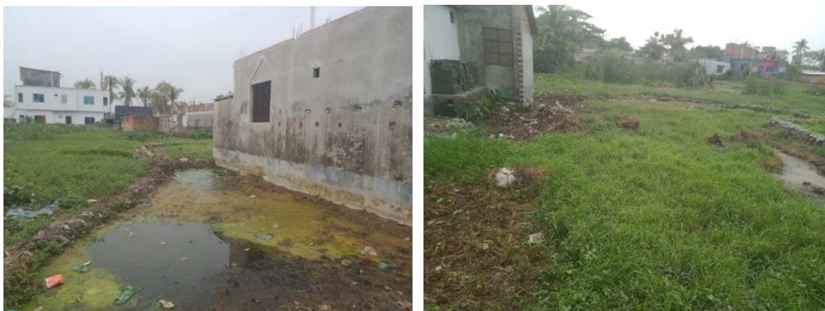
Figure 18: Earthen dyke in the West and North dumping sites
