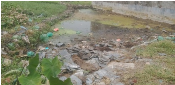
West dumping site before remediation work
