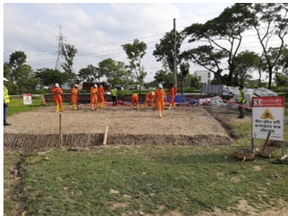
Figure 42: Filing south dumping site with 1 ft excavated sand and 1ft clean soil.
