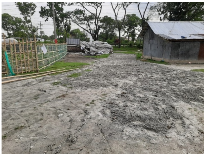
Figure 54: Unpaved area damaged due to the heavy vehicle transportation was repaired.
