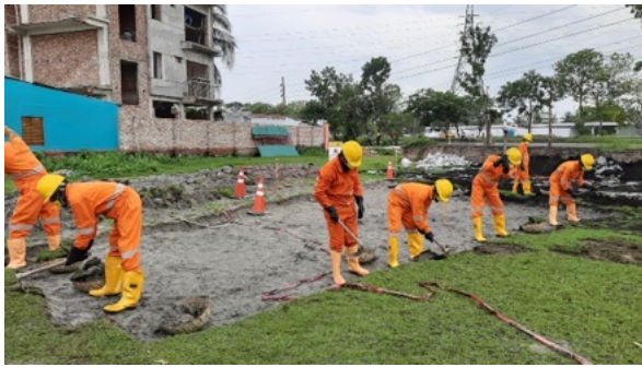
Figure 36: Excavation of top 1 ft soil of the south dumping site.
